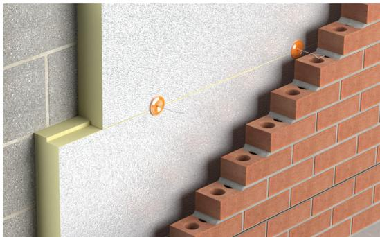
5. Ensure a minimum 225mm overlap with the floor insulation. The receiving block should be plumb to provide a flat surface to accept the insulation. As with setting out, installation should commence from adjacent corners using the Cavity Wall pre-formed corner boards. Alternate corner boards will achieve the offset break bonded pattern for the insulation.
